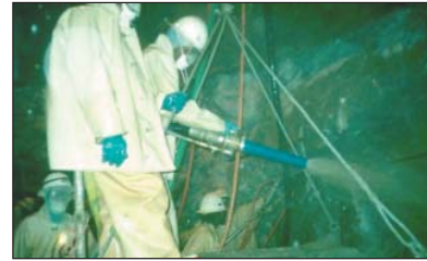
Shotcreting in progress.
