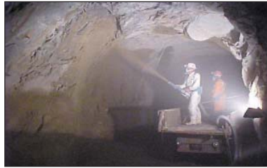
Shotcreting in progress.
