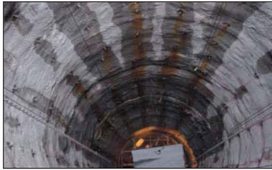
First layer shaft concrete.
